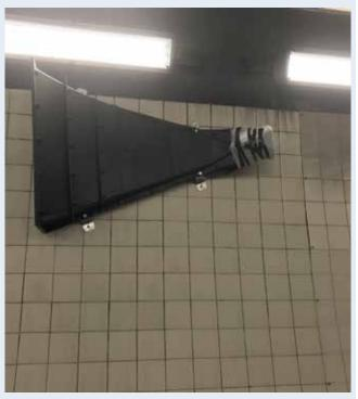
One of the wall mounted speakers for a new public address system to improve communications inside the Lyttelton Tunnel. The system broadcasts safety instructions to tunnel users in an emergency.
