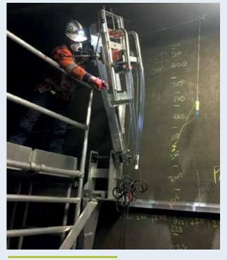
The working platform and drill rig designed for ensuring tunnel duct panels loading restrictions and increased hole drilling efficiencies are achieved during the installation of 9km of new pipe, held in place by 1326 brackets. Crews often have to walk up to 1km to reach their work site inside the tunnel ducts dressed in full protection kit – not an easy task.
