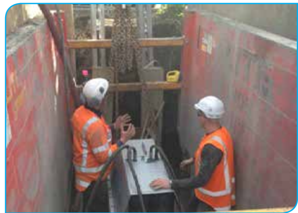
The pulling unit inside the exit trench
