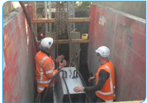
The pulling unit inside the exit trench
