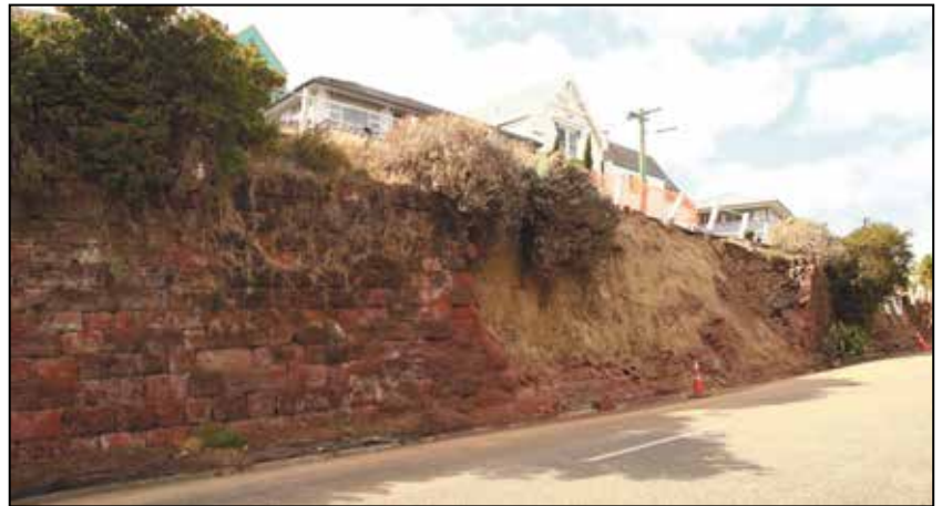
Example of damaged red brick retaining wall in Lyttelton
