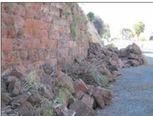
Example of damaged red brick retaining wall in Lyttelton
