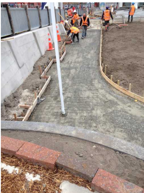
Boxing and reo ready for concrete
