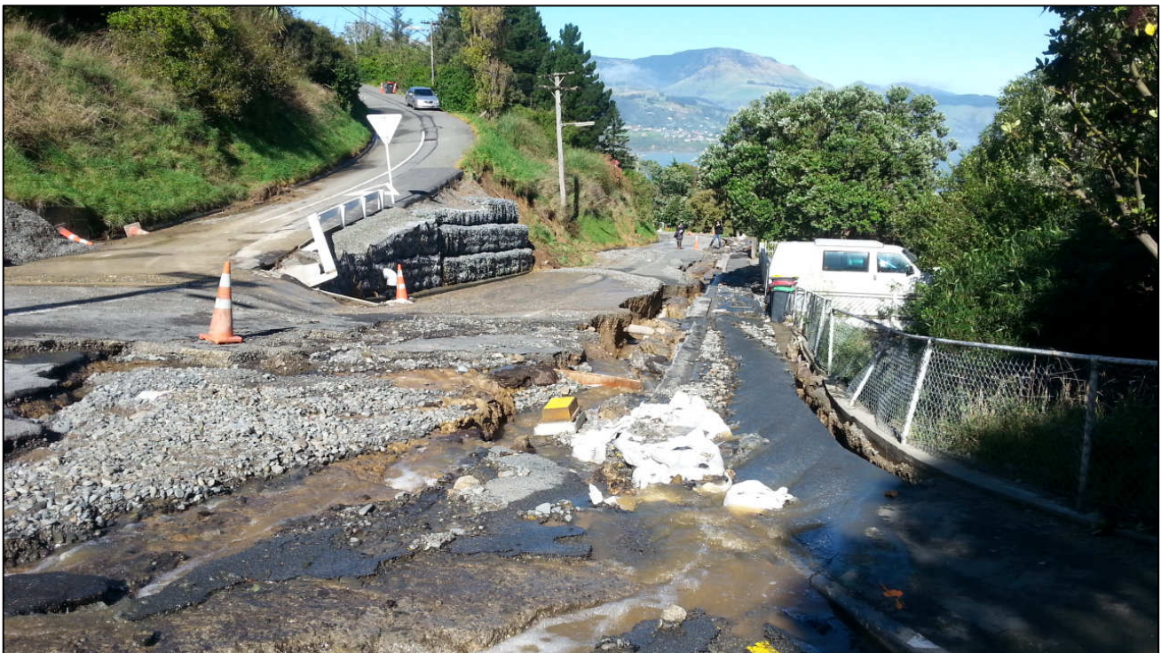
Caption: Flood damage in Canterbury Street after the April rains this year.
